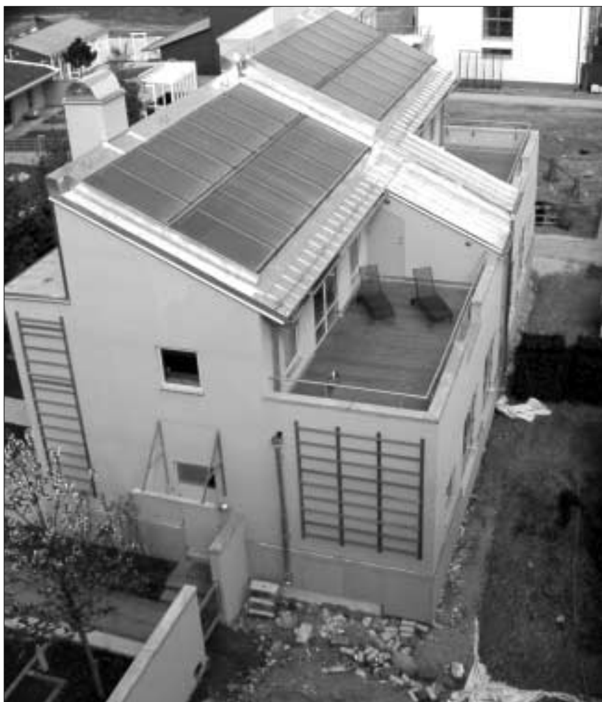
In the City of Tomorrow (Malmö, Sweden) 120 m 2 of photovoltaic cells help supply energy needs
