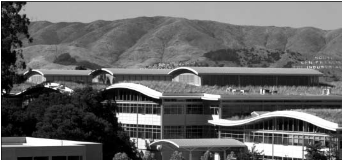
The roof of 901 Cherry (offices of Gap, Inc.) recreates the native habitat of grasses and wild flowers. Its form derives from the surrounding landscape. © William McDonough + Partners
