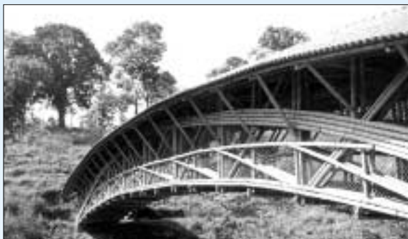
52 metre bamboo road bridge by Jorg Stamm (Colombia) and bamboo scaffolding (Hong Kong)
