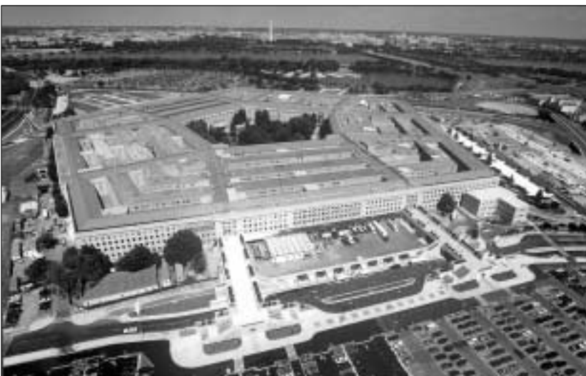
Pentagon renovation project in Washington, D.C.
