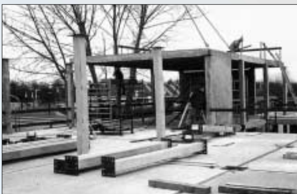
Dutch MXB-5 system: reinforced concrete buildings can be dismantled and reassembled at new locations, as dictated by government policy and economics
