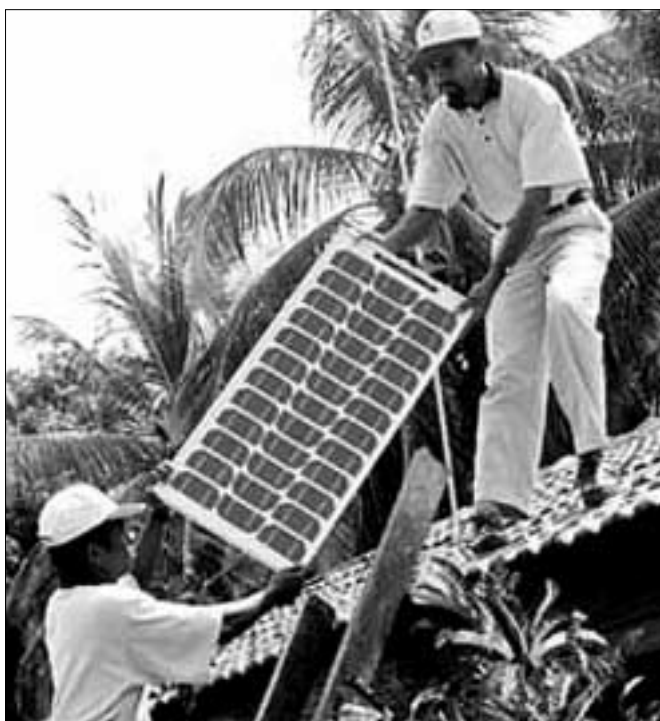
Installing a solar home system
