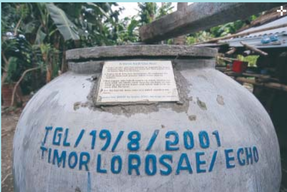
Figure 6-3: A placard, which describes the operation and maintenance procedure for a family to follow, is attached to each rainwater jar.
