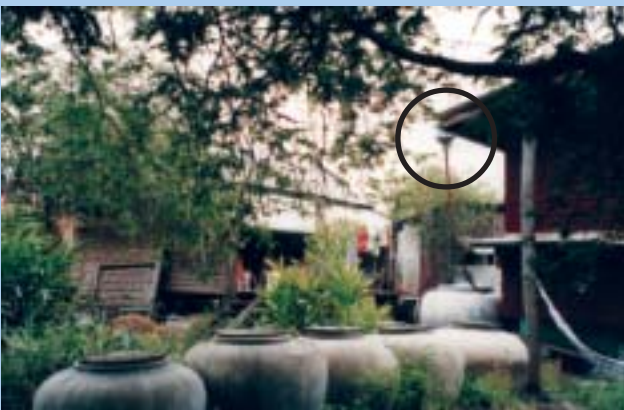
Figure 5-6: A piece of plastic tube attached to a funnel hanging under the gutter outlet is used as a connecting pipe. The plastic tube can be moved away from the mouth of the jar or the tank inlet to drain away the first and the second rain of the season.
