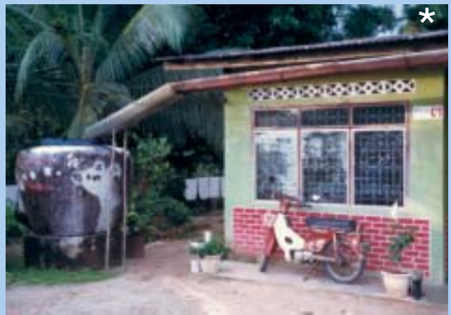
Figure 5-5: A piece of galvanized sheet bent into a "U" shape is used as connecting pipe for rainwater to flow from gutter outlet to the jar.
