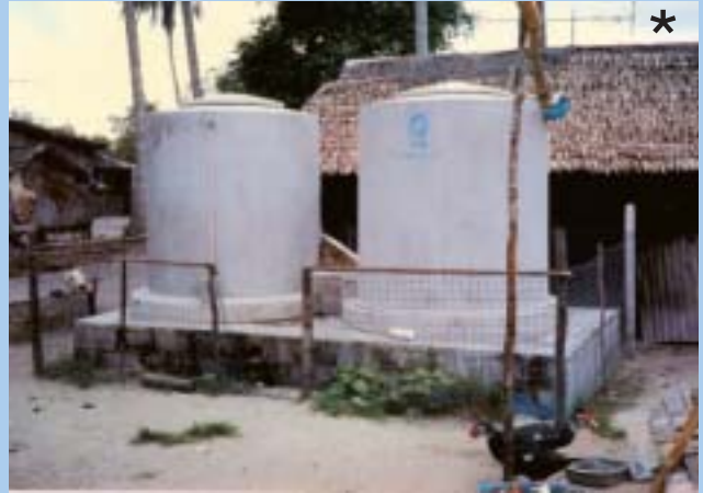
Figure 5-3: Bamboo is used as connecting pipe between the gutter outlet and the inlet of the tank.
