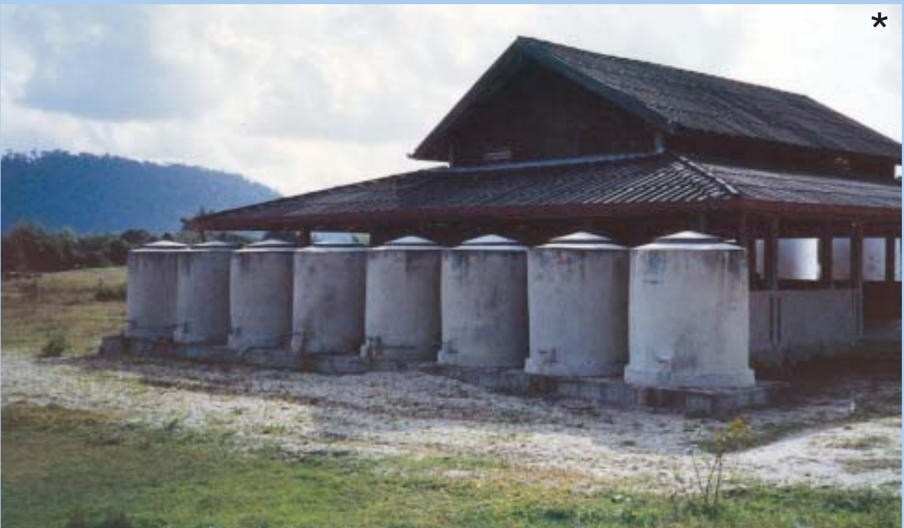
Figure 5-16: The rooftop of a village meeting place is an idea rain catchment. Series of tanks are installed on the ground to collect rainwater from the rooftop for community consumption.
