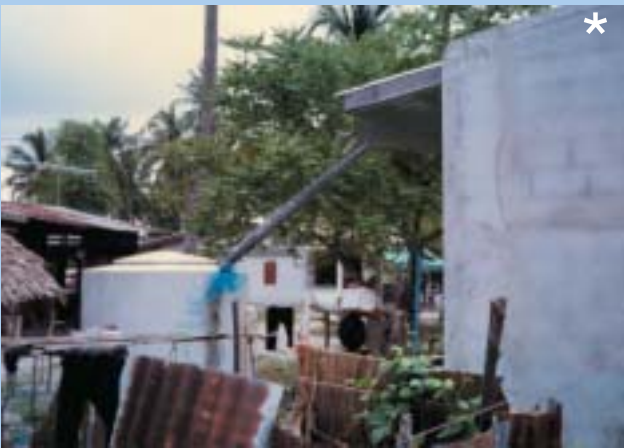
Figure 5-4: A piece of galvanized sheet bent into a "U" shape is used as connecting pipe for rainwater to flow from gutter outlet to the tank.
