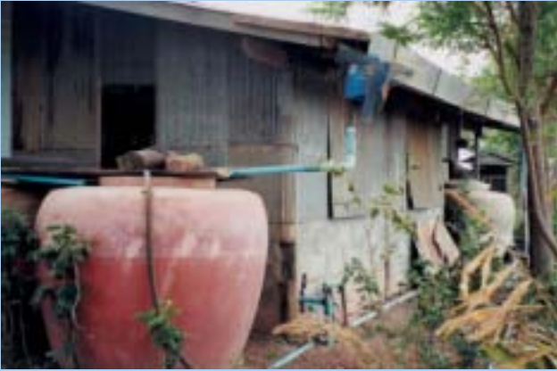
Figure 5-8: A plastic bottle is used in replace of the funnel and fixed onto the connecting pipe inserted into the mouth of the jar.
