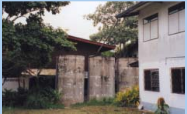
Figure 5-11: This household shows an innovative way of making three rainwater tanks with very large diameter cement rings to store rainwater collected from the rooftop.
