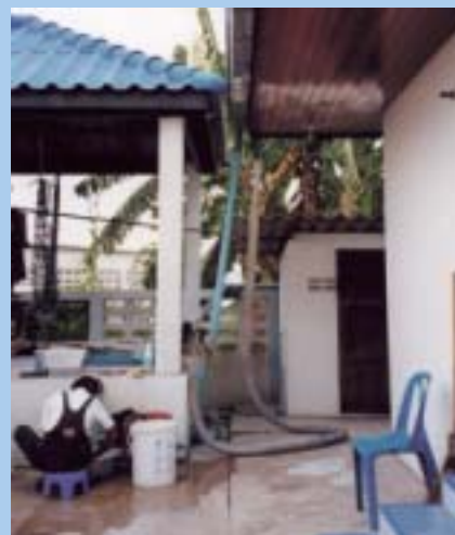
Figure 5-13: Household collects rainwater from rooftop, which is stored in a square tank built on the ground. The connecting pipe between the gutter outlet and the ground tank is a plastic tube.
