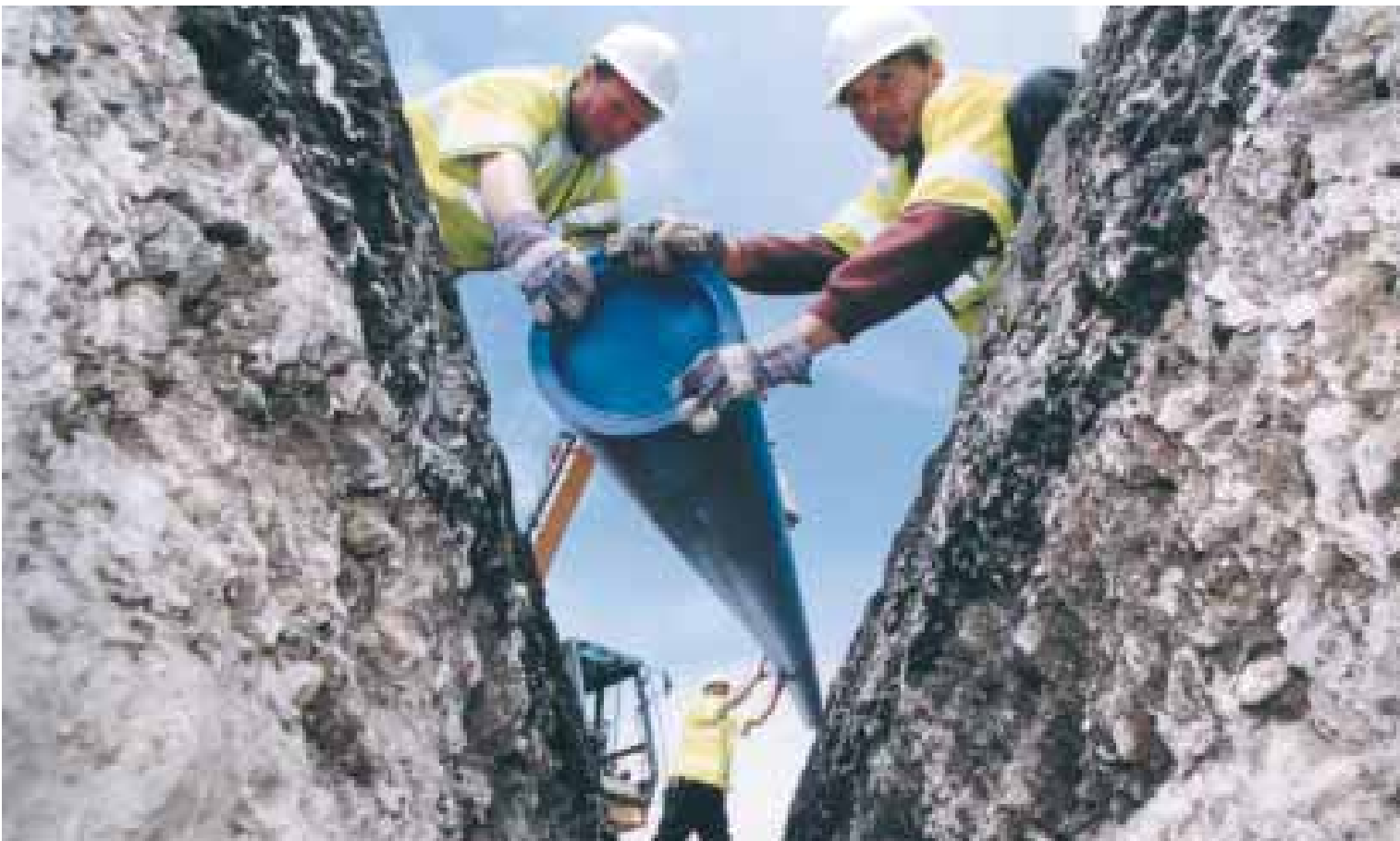
Installing water supply pipes in the Thames Valley, UK
