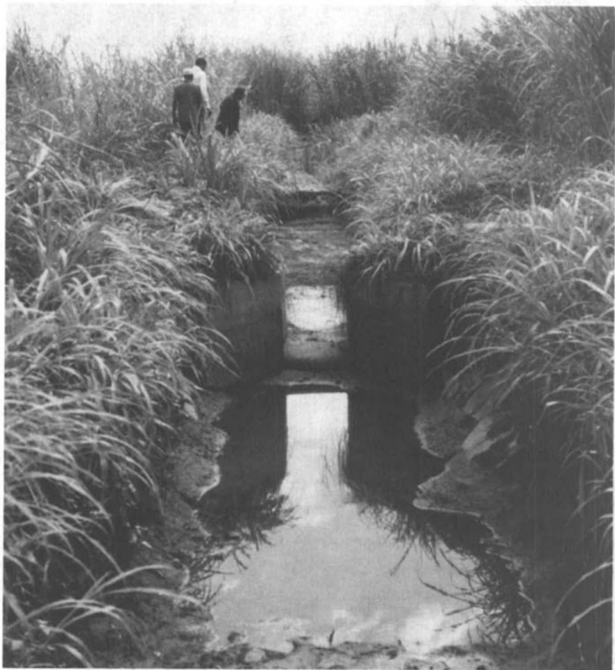
Upstream deforestation increased flood flows and silt loads, destroying these irrigation canals in Tanzania.
