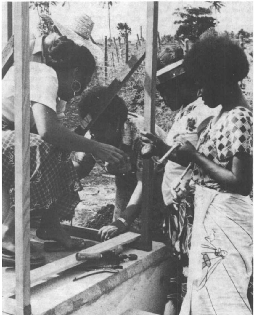
Building the walls of the latrine.
