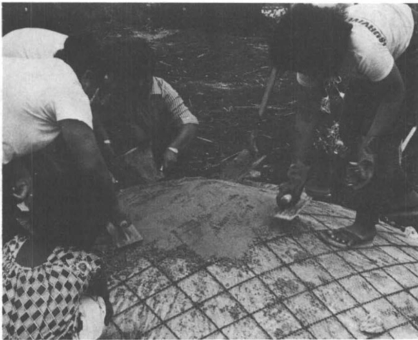
Reinforcing the top of the VIP latrine.
