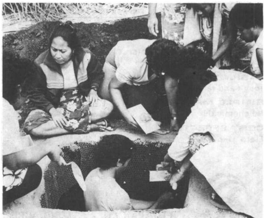
The ferrocement water tank is reinforced with chicken wire.
