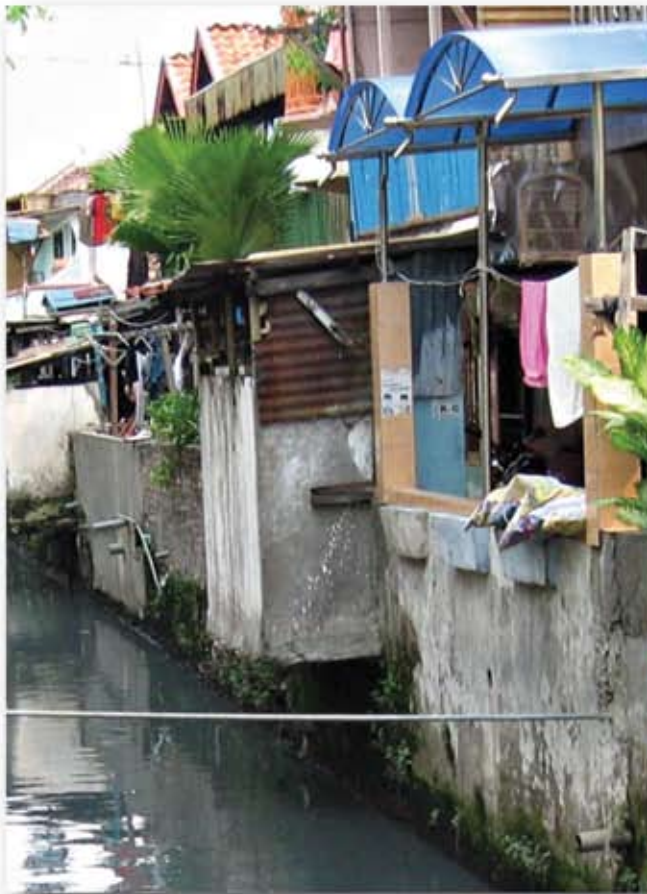
Regulations must strictly prohibit dumping of raw sewage in rivers. Helicopter latrines like this one should not be allowed.
