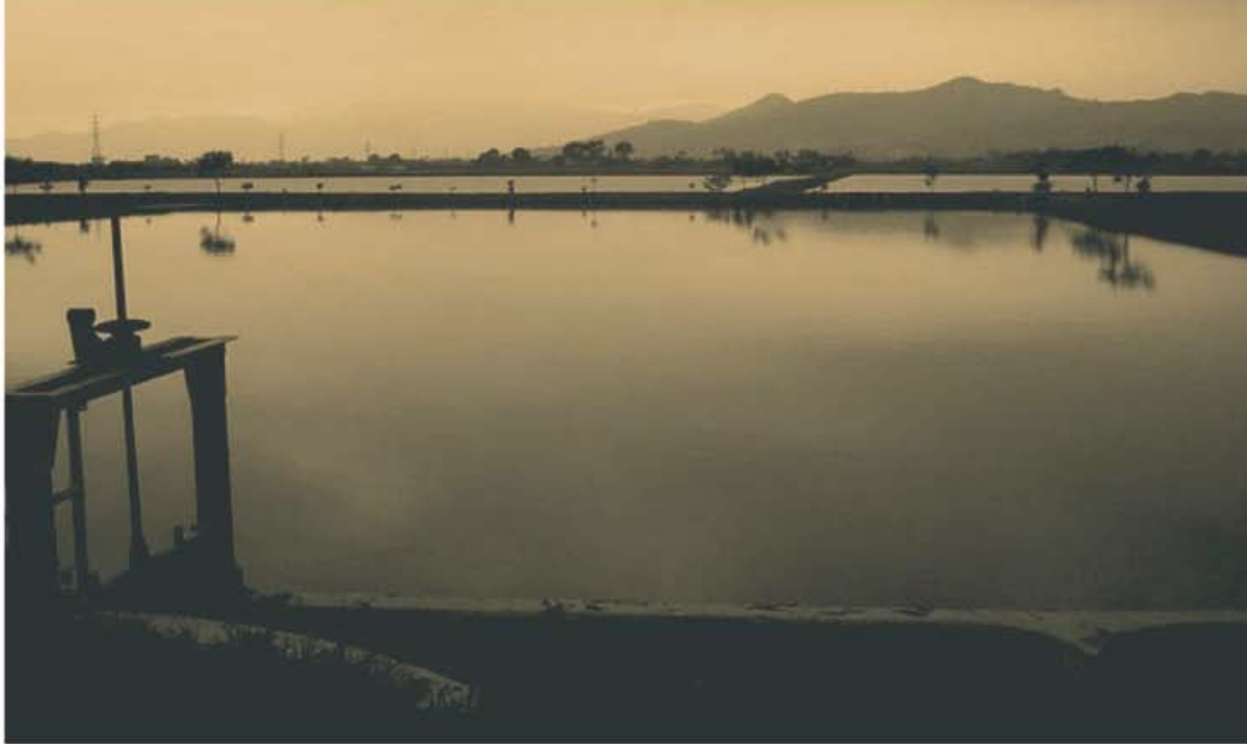
The sewerage system in Bandung uses the simple treatment technology of oxidation ponds. In the near future, the Bandung city water utility, which manages the system, will be installing aerators in these ponds. Eventually, the sewerage system in Bandung should be able to offer a better service to 40% of the city's population.
