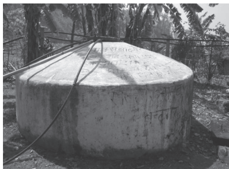
ADB Water Tank
