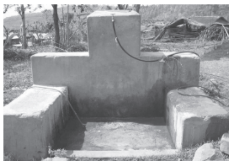
Private pipes allow locals to bring water right into their back yards.
