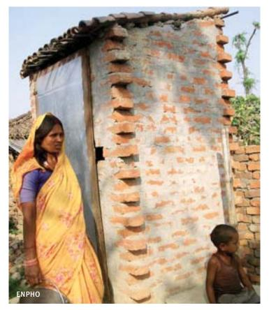
of EcoSan toilet, the urine is collected separately while the faeces, together with the water used for anal cleansing and flushing, is collected in a pit. Except for the pan, where two separate holes are provided for urine and faeces, and the urine collection pipe and tank, all the components of
