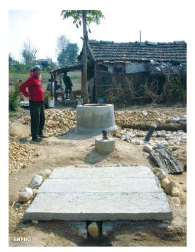
Photo 2.4: Newly constructed biogas plant with inlet for toilet
