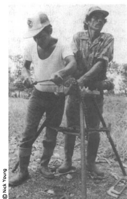
Installing a handpump.
