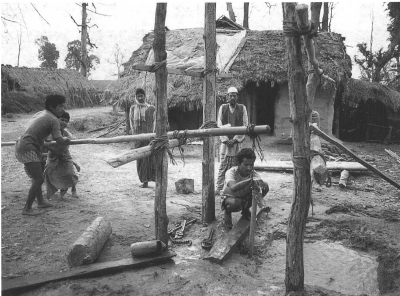
A Nepali mistri covers the pipe with his hand to create a vacuum, while the assistant operates the bamboo lever.
