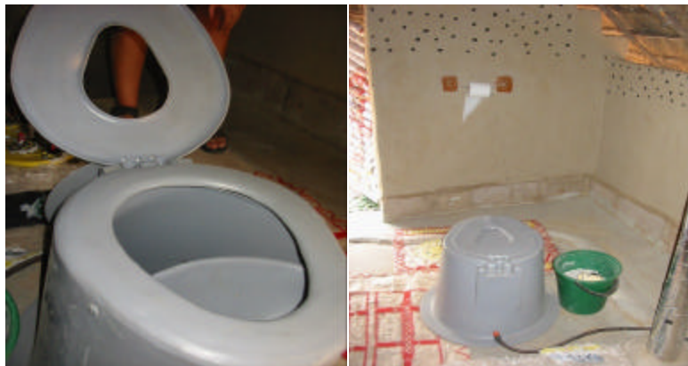
Urine diverting pedestal alone (left) and in the toilet with bucket of ash (right)
