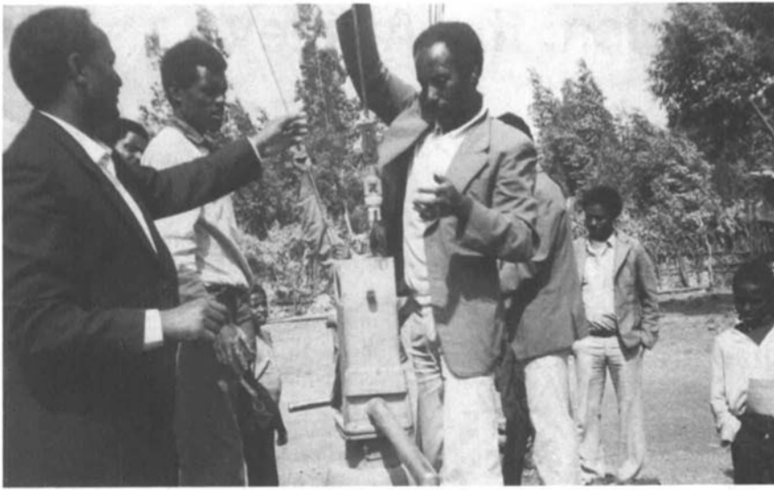
A handpump caretaker learns how to remove a footvalve from an Ibex Afridev in Asgori, Ethiopia.
