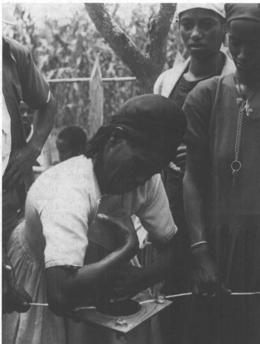
The women of Lamarada have become handpump caretakers and are installing their own Afridevs.
