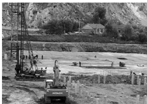
Hailin Waste Water Plant ©SHP
