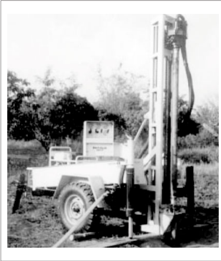
Figure 10: ACF-PAT 301 T. Rig in drilling position.
