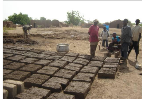
Photograph 4. Brick moulding at dam site
