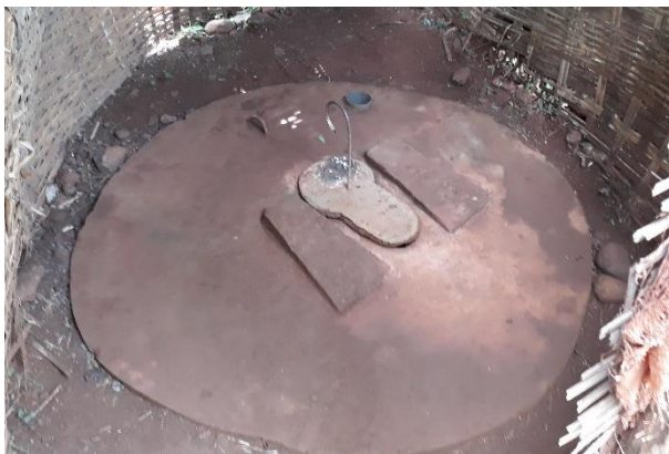
Pre-cast circular concrete slab (120 cm) with removable drop-hole cover
