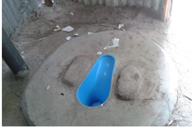
SATO pan with concrete skirting
