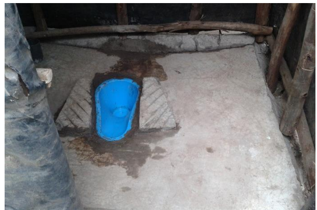
Pre-cast rectangular concrete slab (120 x 120 cm) with SATO pan
