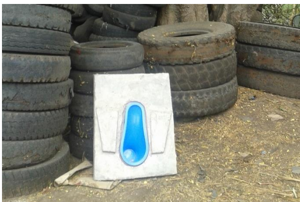
Pre-cast concrete mini-slab (60 x 80 cm) with SATO pan
