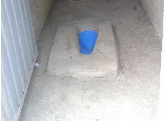
SATO pan with concrete skirting
