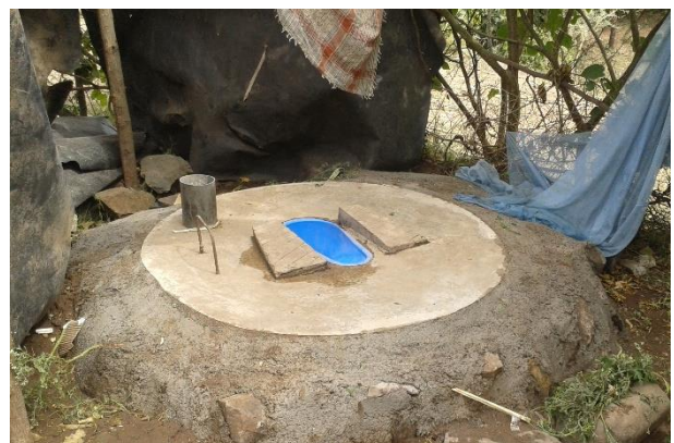
Pre-cast circular concrete slab (120 cm) with SATO pan
