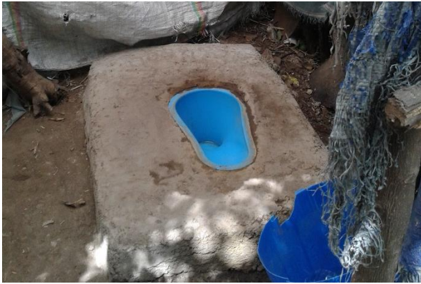
Retrofit of SATO pan on wood/mud slab
