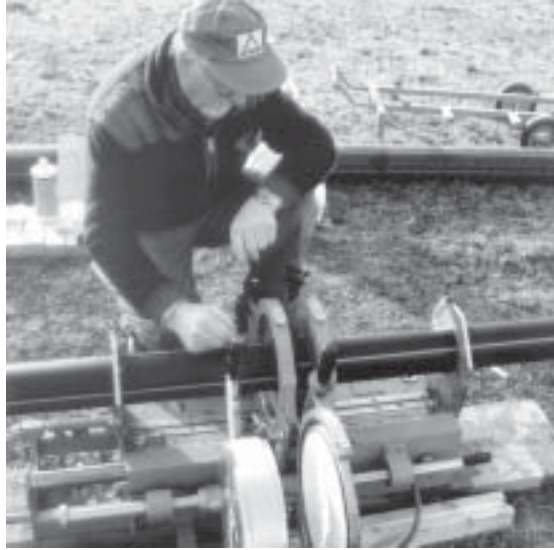
A one man enterprise specialised in welding of PE pipes an house installations
