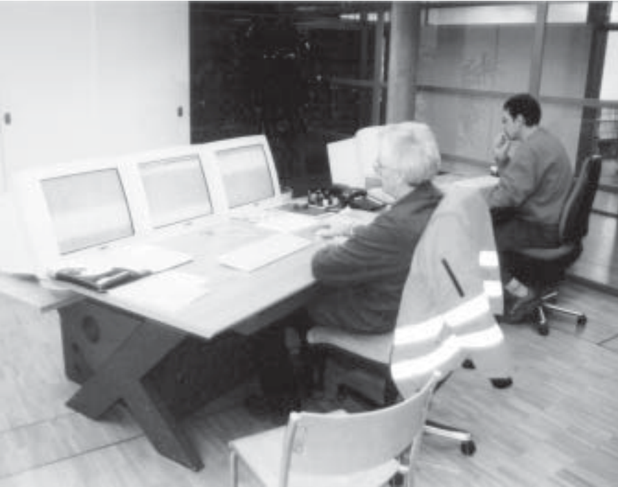
The caretaker checking the network electronically. All the pumps and reservoirs are monitored by a computer network.
