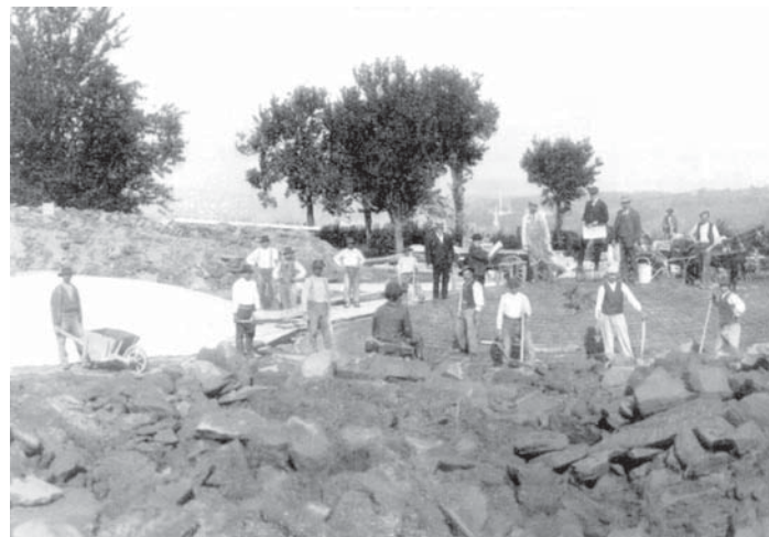
Construction of the two main reservoirs in 1913 - a labour-intensive process involving many of the village men.
