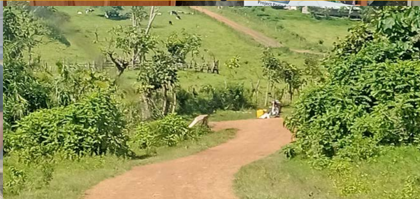
Status of Harugongo - Kakundwa - Busoro community access Road
