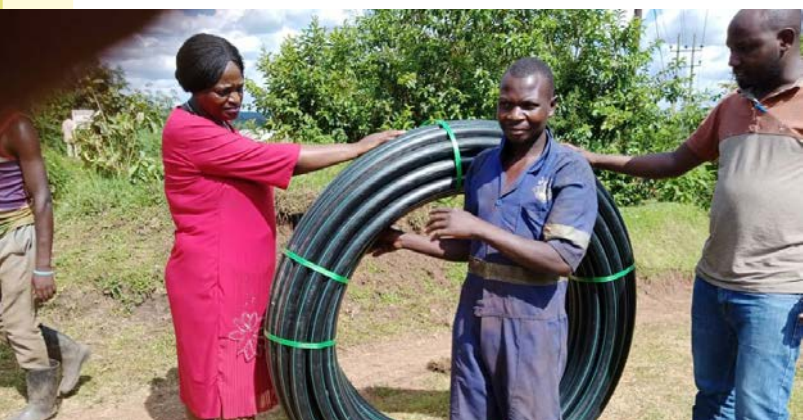
Extension of piped water in Kyamazima.
