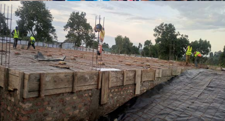
Latest status of Kihondo marketshed in Kichwamba sub county Kabarole district
