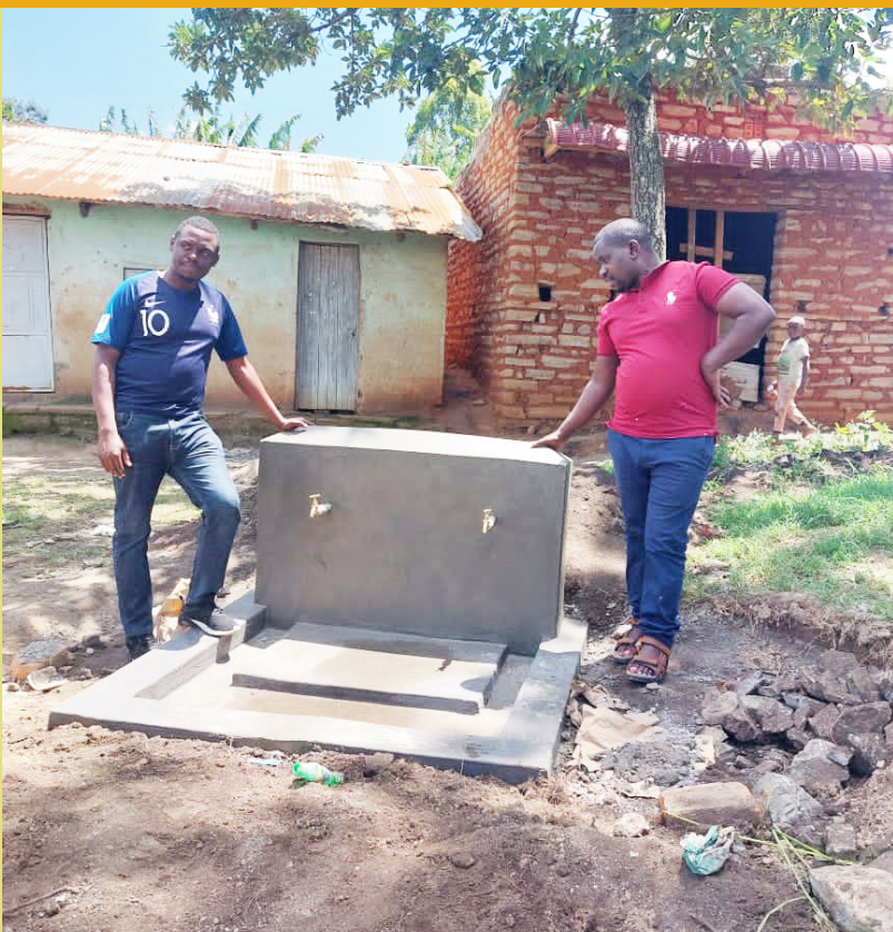
Extra works of extension in Kagogo village
