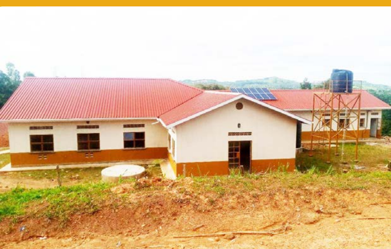
Ruteete maternity ward constructed by World Bank
