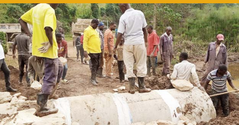
Installation of culverts on Ruteete Mituli road
