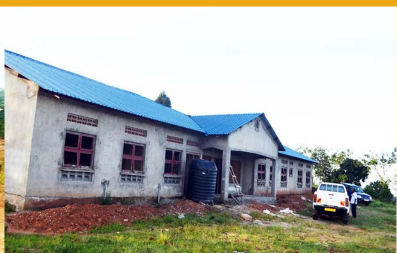
Construction of Kitule Health Center III Maternity ward
