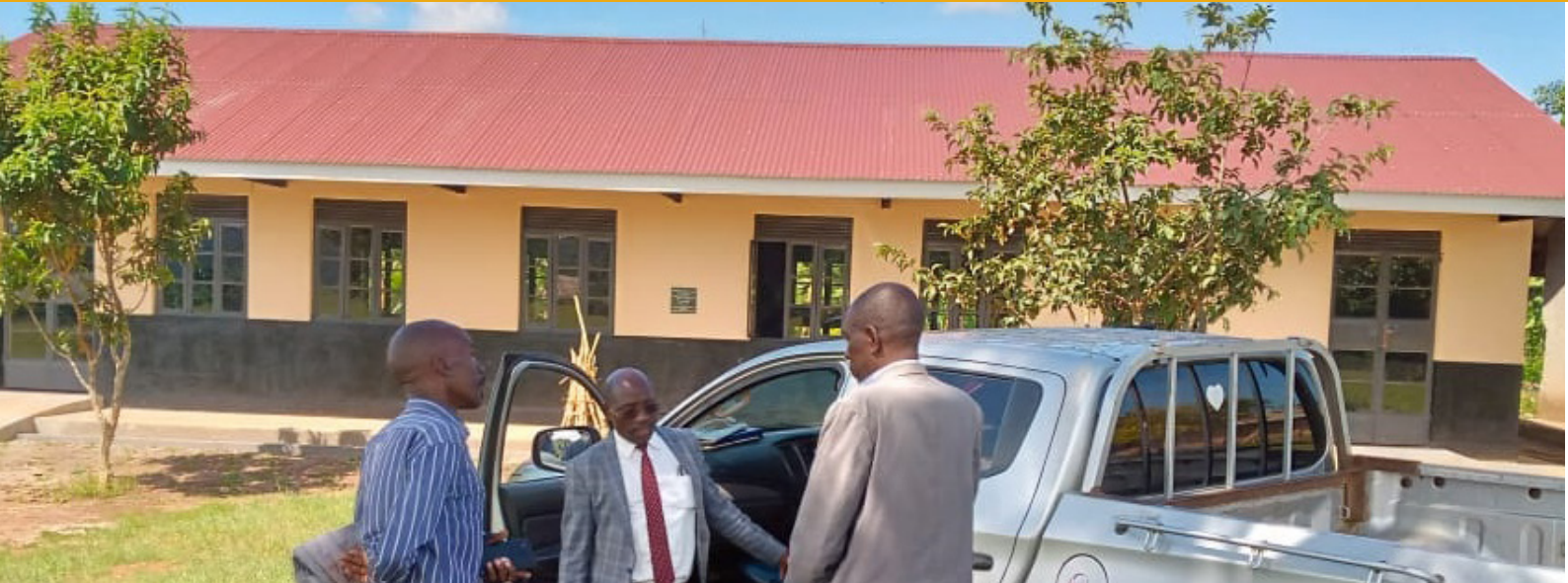
DEO and chairman school management committee monitoring Bunyonyi primary Kibasi Town Council that was constructed this financial year
