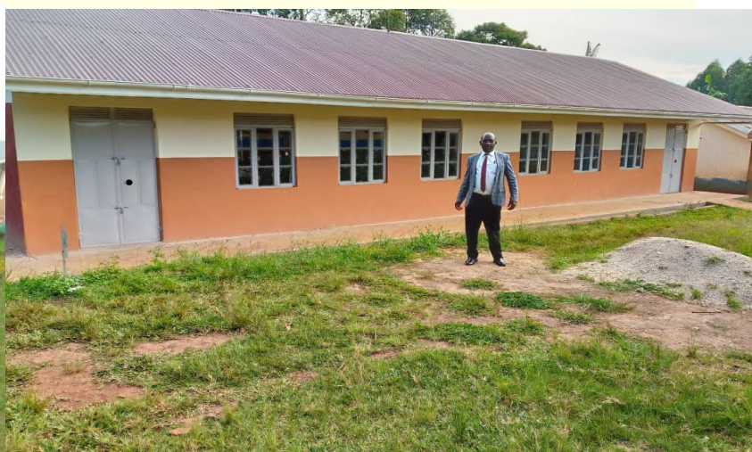
Mr. Rujumba Joseph Ag. DEO monitoring construction of a classroom block at Kyanyawara Primary Kiko Town Council
