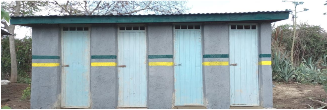
Figure 5: School sanitation facility. Photo credit: BBBC Negelle Arsi field office
