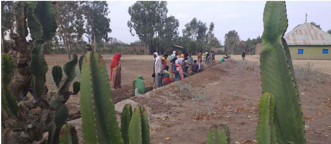
Figure 1: Community working on trench excavation and backfill. Photo credit: Amref
