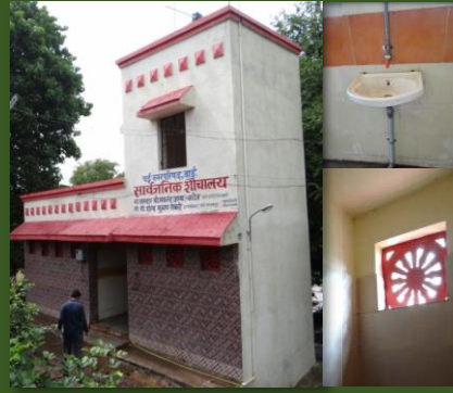
Community toilet at Wai. Provision of wash basins, room for care taker.
