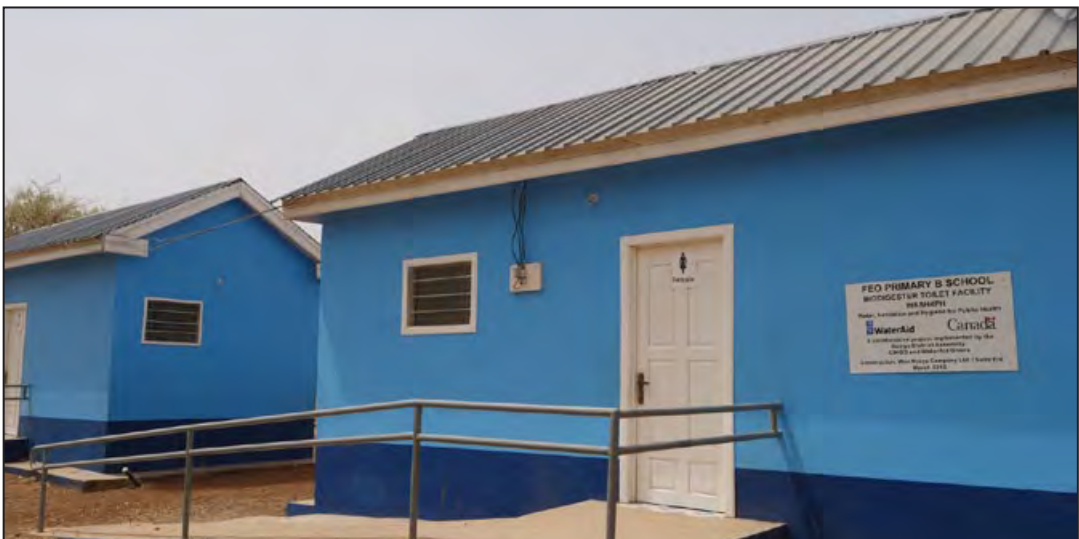
Modern flush toilets with menstrual hygiene facilities at Foe Primary School B, in Bongo District
