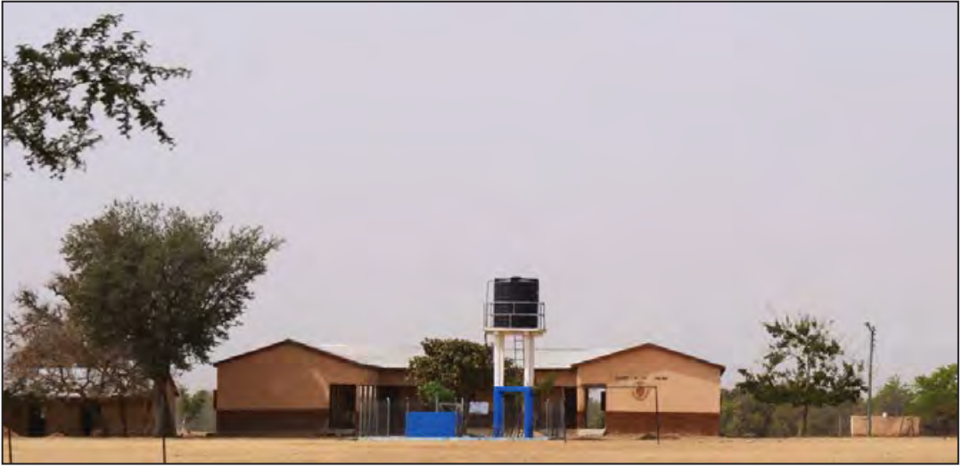
Mechanised systems with solar technology avoid the need for electricity bills for pumping water .
