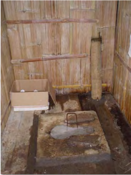
Example of a locally produced sanplat model purchased by a rural household, Commune of Ambodimangavalo
