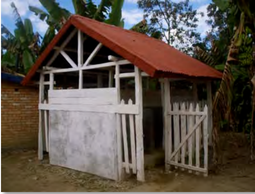
Example school latrine with separate cabins for boys and girls built with local funding from a parents association in the commune of Beforana
