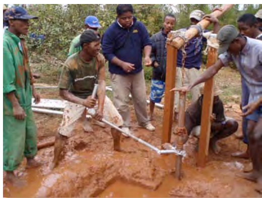
Training 4 NGO in the Rota-sludge manual well drilling technique
