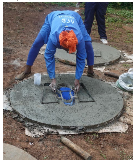
Woman installing SATO Pan (Picture Credit: PSJ)
