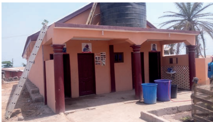
This 24-seater public toilet facility in Yeji takes into consideration the needs of vulnerable groups in the community.
