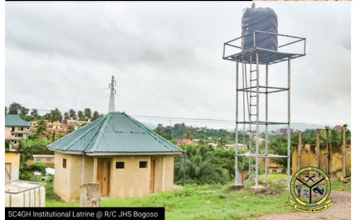
SC4GH Institutional Latrine @ R/C JHS Bogoso
