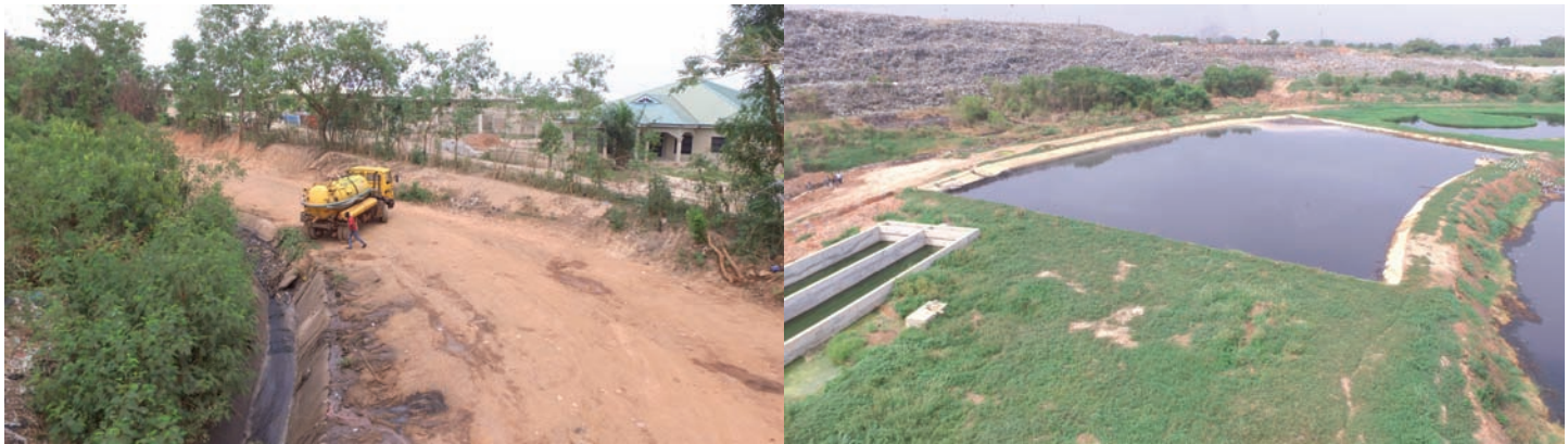
Oti anaerobic pond before (left) and after (right).
