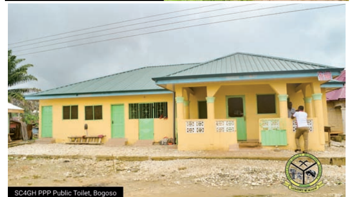
SC4GH PPP Public Toilet, Bogoso
