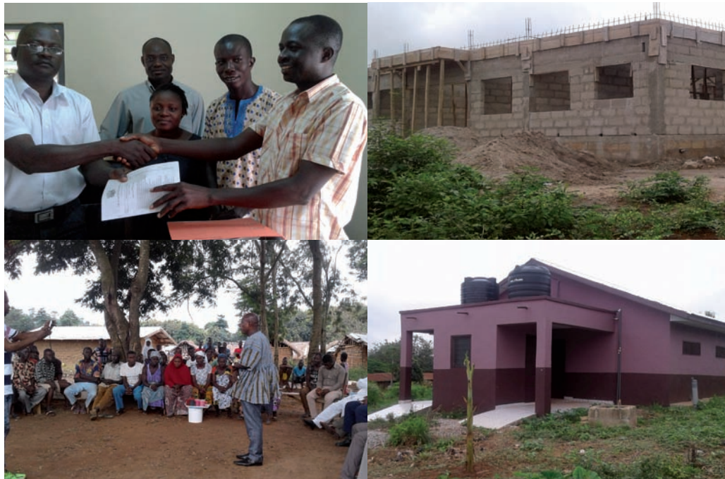
A copy of Da by-laws being presented to management of the Assembly (top left), construction of a 20 -seater W/C toilet facility in Akomadan Timber Market (top right), DCE addressing community members on sanitation issues during community durbar at Sarfokrom (bottom left), and a completed 10-seater W/C toilet facility in Akomadan English-Arabic (bottom right)
