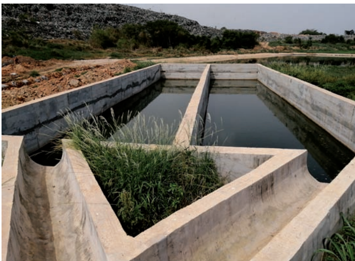
Oti settling tank
