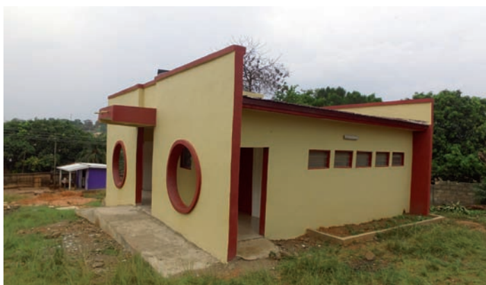
Adumanu School latrine
