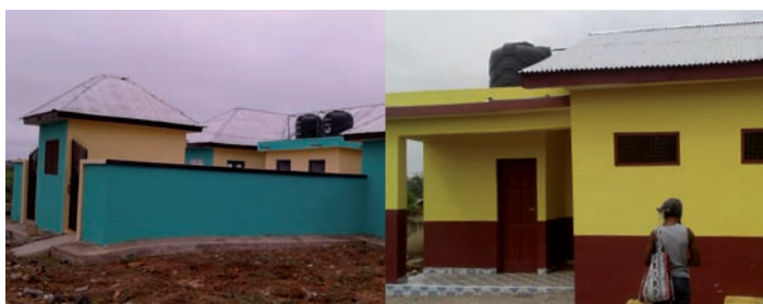
Completed 20 seater toilet facility in Akomadan - Agric (left) and completed 10 seater toilet facility in Akomadan - Zongo (right).
