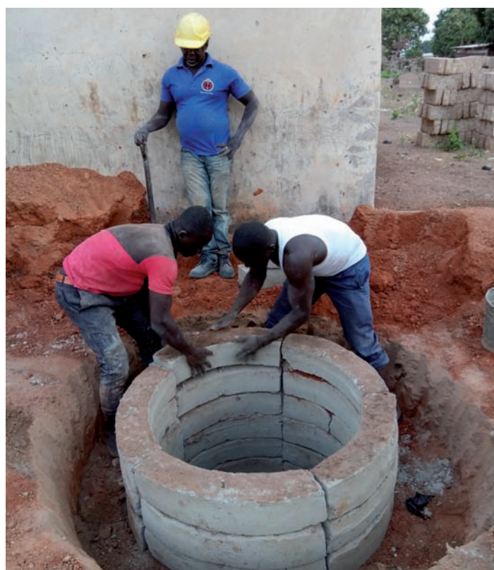
Construction of Circular APDO eco-Safe Toilet for Vulnerable Person in Bimbilla
